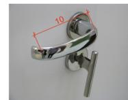
**DETALHE MAÇANETA PORTA: TRINCO DE ALAVANCA ARREDONDADO (COM CHAVE ADAPTADA)**
